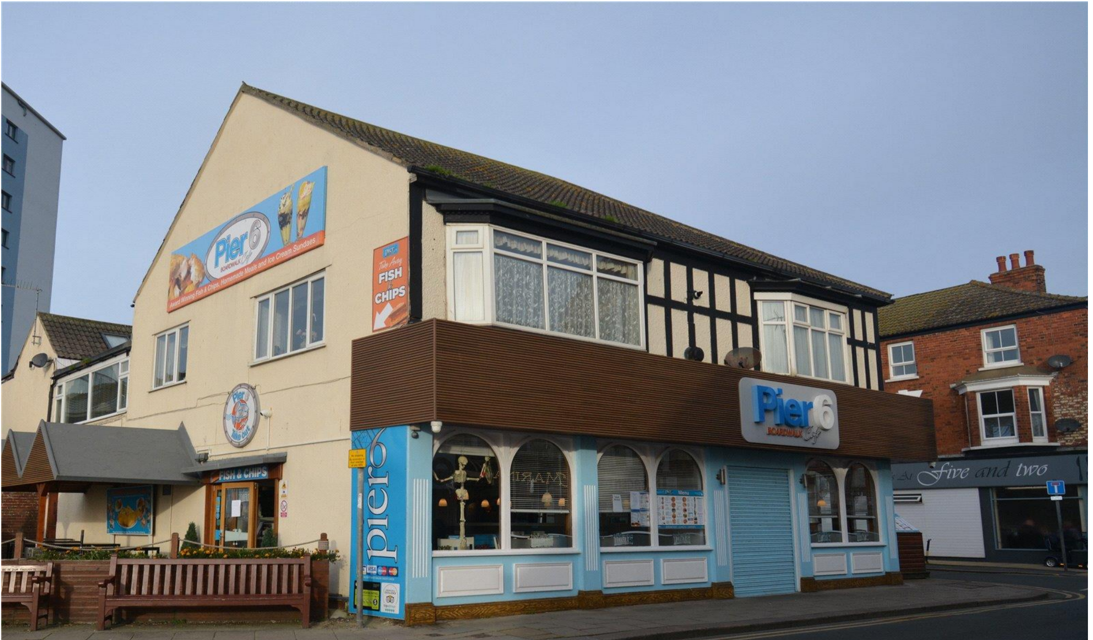
Pier 6, 6 South Cliff Road, Bridlington, EastYorkshire, YO15 3AT
